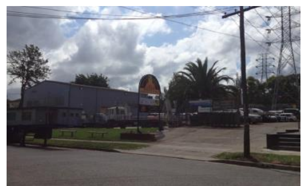
Figure 10. Industrial buildings on Hope Street
