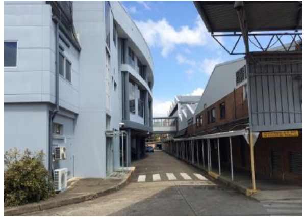
Figure 4. Existing industrial building
