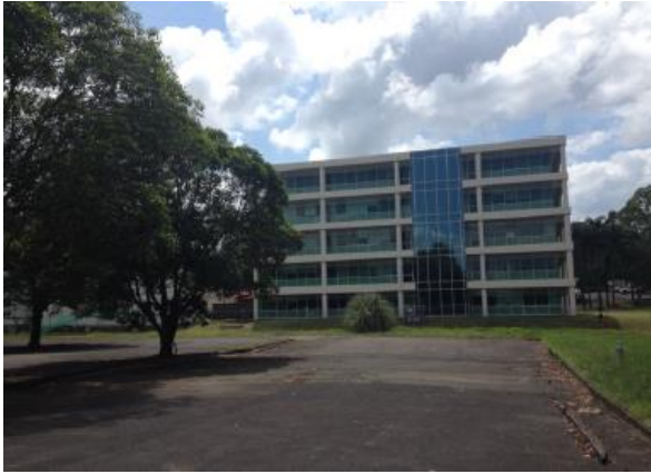
Figure 3. Existing industrial building
